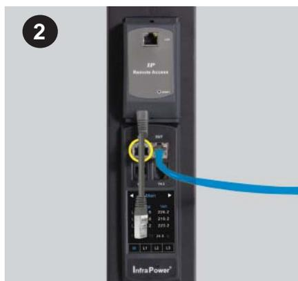
Step 2 - Disconnect the IP dongle jack from the meter
